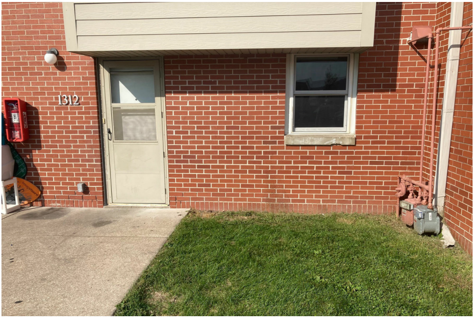
SOFFIT AT FIRST FLOOR WINDOWS
